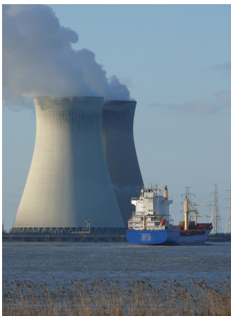
A nuclear power station uses the energy from fission to make electricity; the towers release waste heat as steam
