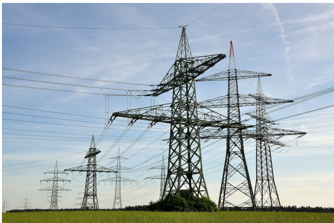
Pylons hold the cables that carry electricity at very high voltage, which keeps the current — and the wasted power — low
