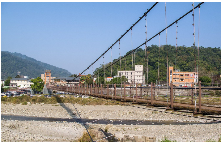
A suspension bridge cable hangs in a parabola — the graph of a quadratic.
