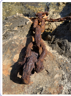
Rusting is a costly form of corrosion
