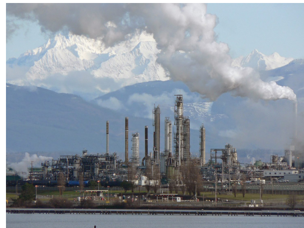
An oil refinery separates crude oil into useful fuels by fractional distillation.
