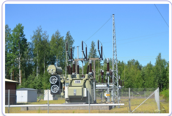
Substation transformer
