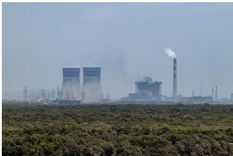
A large utility plant: monopoly and market power mean a single firm can set price above marginal cost
