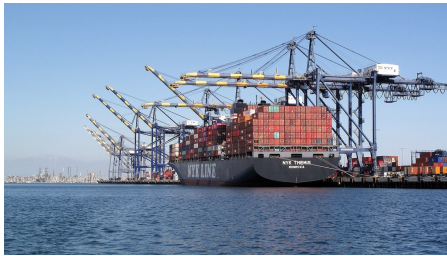
Container ship and cranes, Los Angeles
