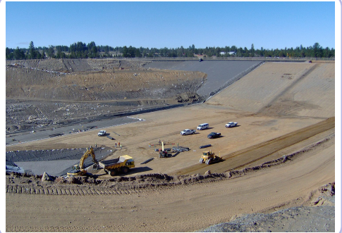
Landfill: line, capture leachate, manage methane
