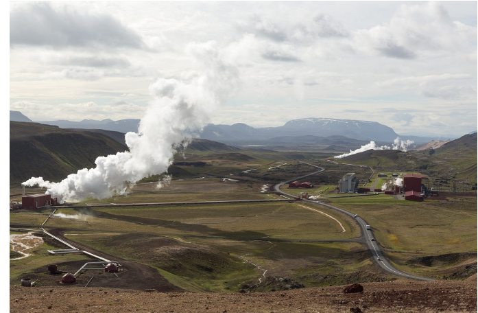
A geothermal power station in Iceland, a volcanic region. Steam 蒸汽 from hot rock below is piped up to drive the turbines
