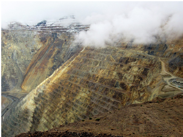
An open-pit mine 露天矿: benches are cut ever wider and deeper to reach the ore, destroying habitat and exposing rock that pollutes water
