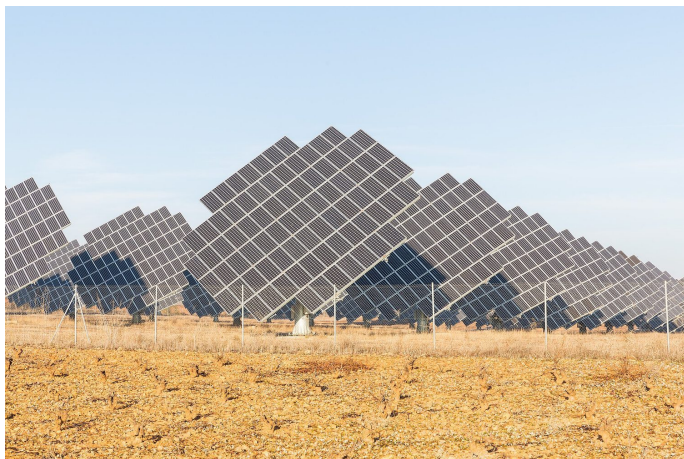
A solar farm: generating more renewable energy and cutting demand are both energy-conservation strategies
