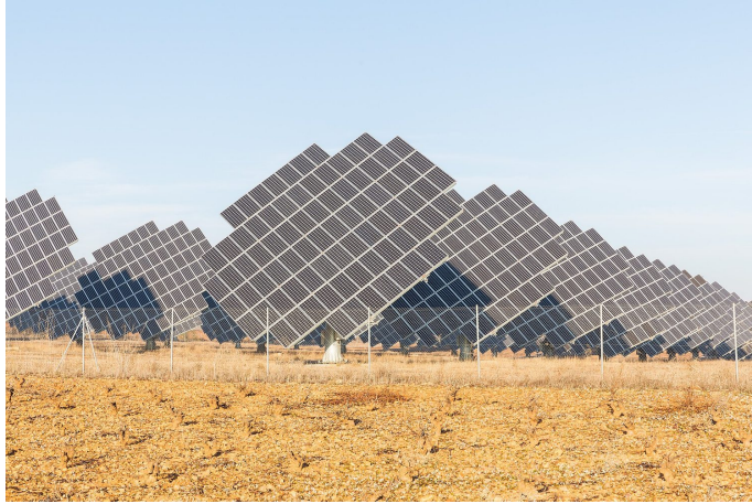
A solar farm. Rows of photovoltaic 光伏 panels are tilted toward the sun; a big output needs a large area of land
