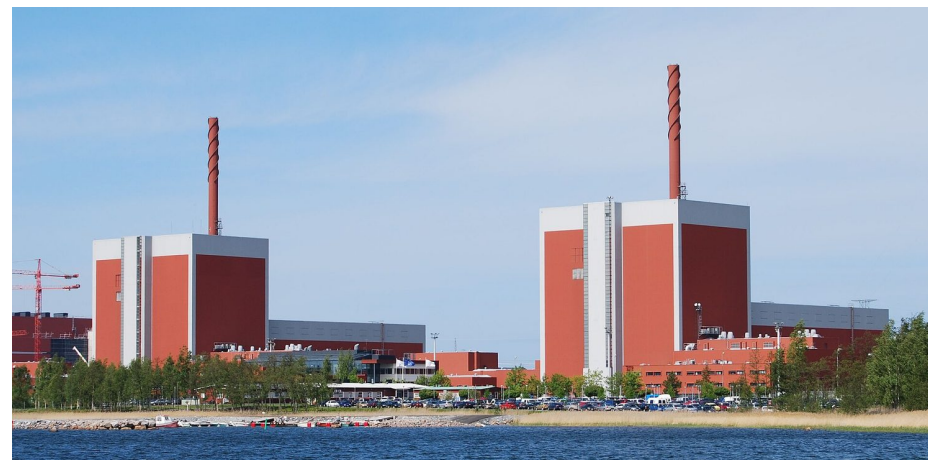
A nuclear power station 核电站. The reactor buildings hold the fuel; the sea supplies cooling water. Notice there is no smoke — fission releases no \text{CO}_2
