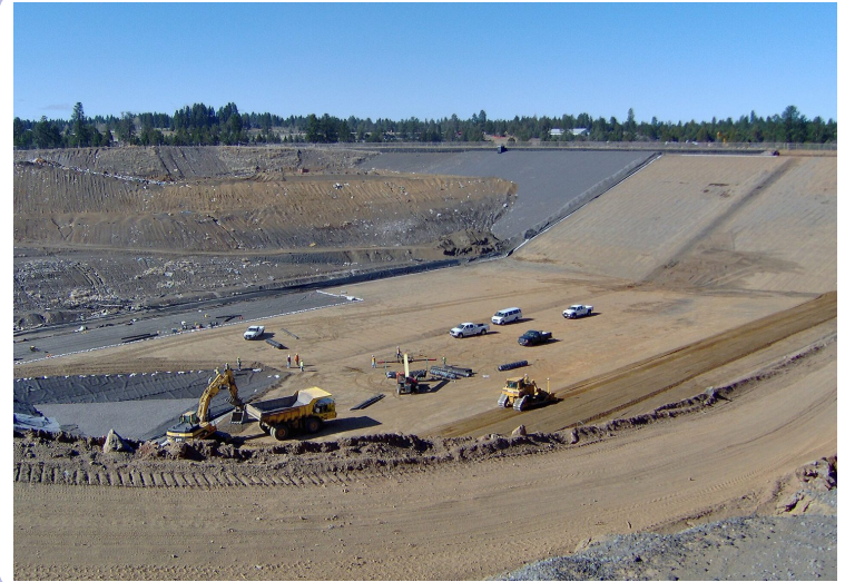
Landfill: line, capture leachate, manage methane
