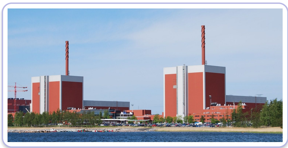
Nuclear: steady low-carbon power, long-lived waste
