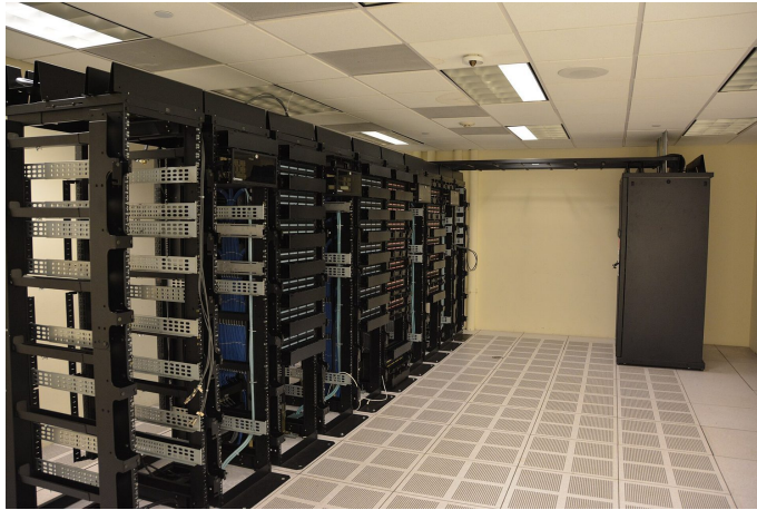
Server racks: network segmentation isolates systems so one breach does not open everything
