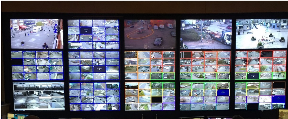
A monitor wall: network monitoring and logging help detect intrusions
