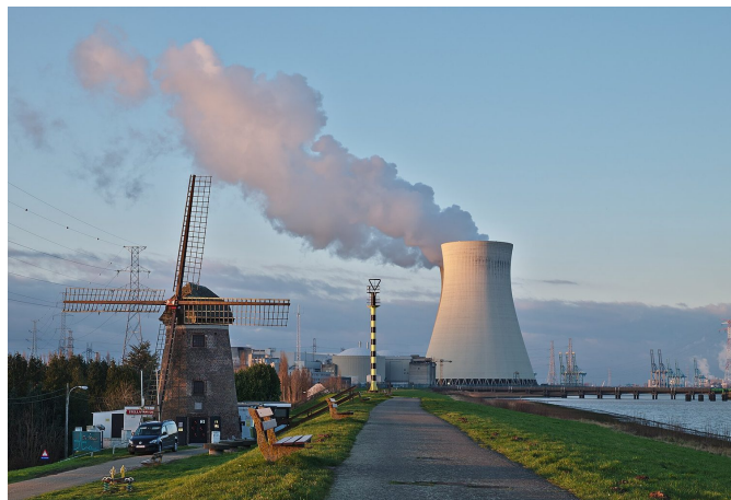
A nuclear power station releases energy by nuclear fission.
