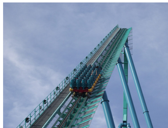
A coaster train hauled up the lift hill: the work done against gravity is stored as gravitational potential energy
