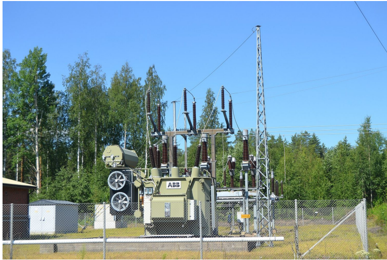
A substation's transformers step alternating voltage up or down.
