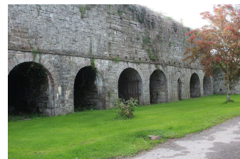
limestone decomposes in a kiln
